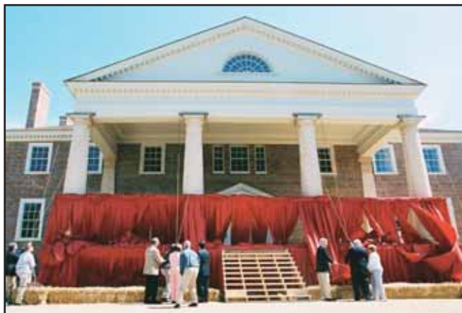
John F. Macon helps to pull ropes revealing the restored portico. Photo by Richard Robertson, courtesy of the Montpelier Foundation.
